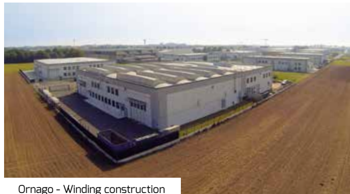
Ornago - Winding construction
