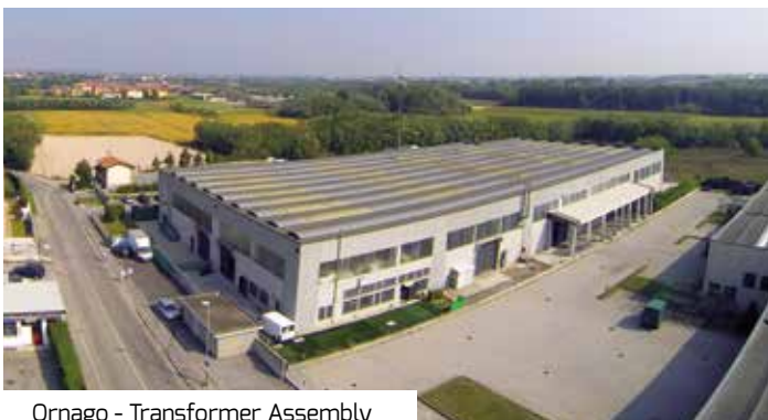
Ornago - Transformer Assembly
